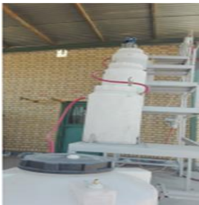
Figure 1. Stair and Tank
