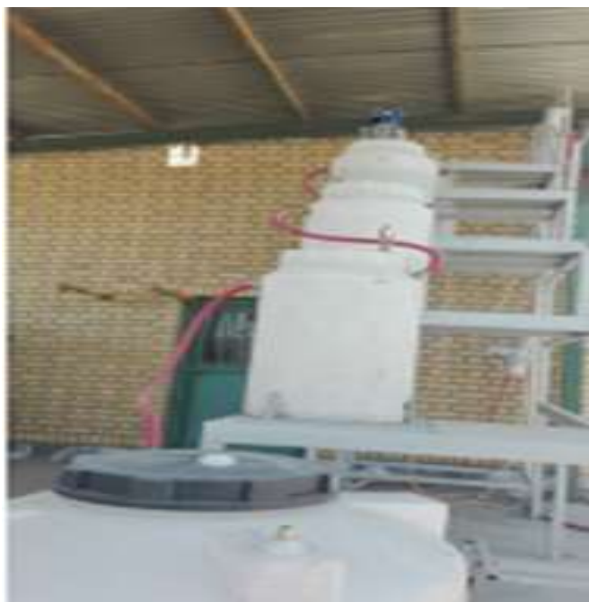
Figure 1. Stair and Tank
